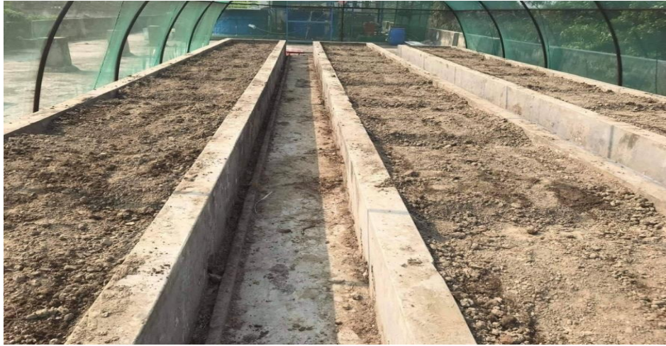
Plate 2. Rooftop land structure
